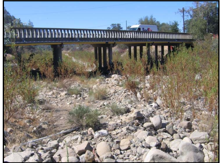
View downstream at the Grand Ave. bridge
