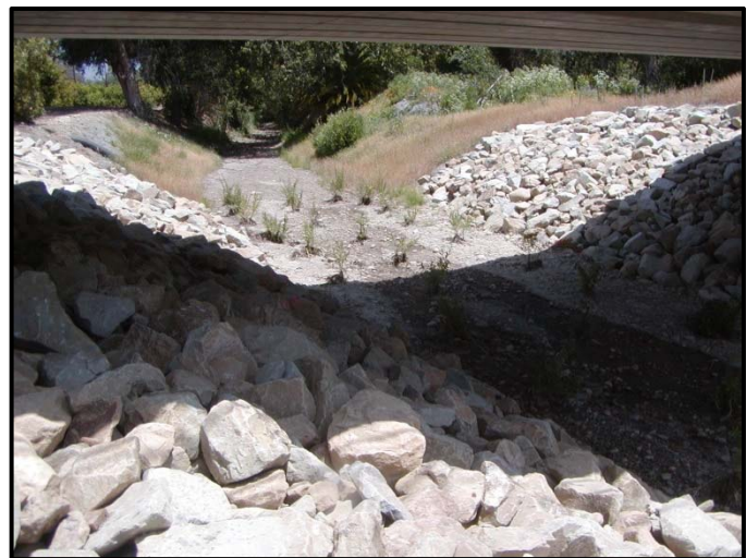
View upstream at the bridge
