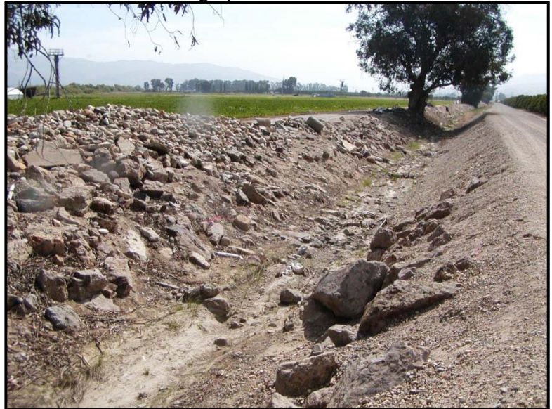
View of site looking upstream
