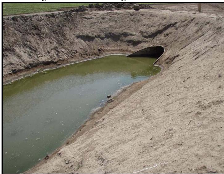
View toward S looking downstream on ag drain before the culvert draining into Revolon Slough
