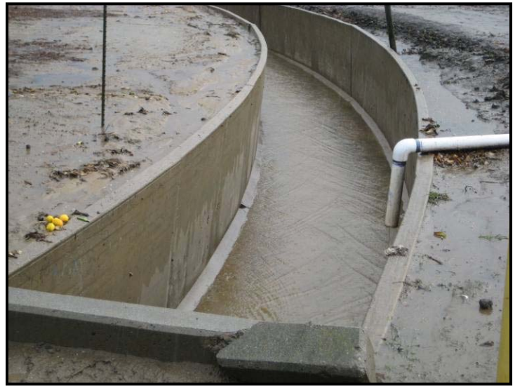
View upstream (NE) from sampling location
